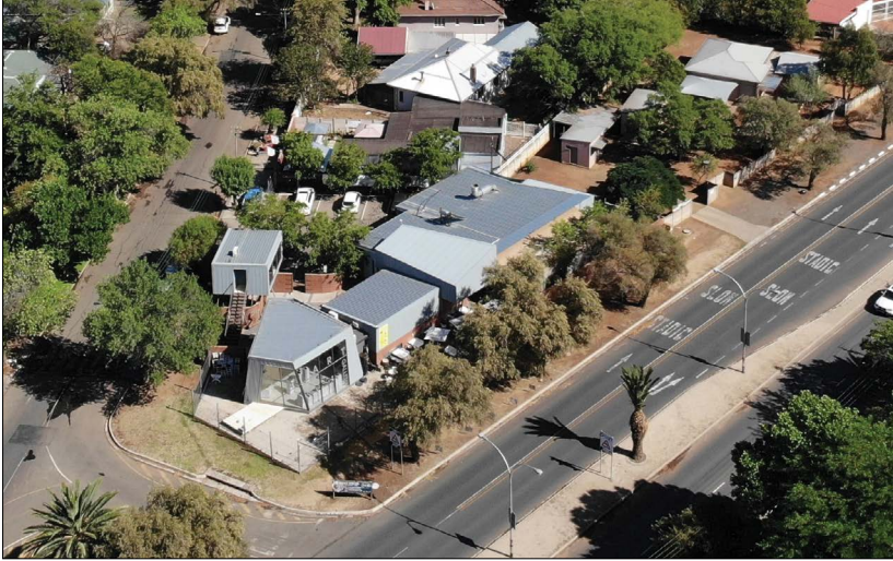
Fig. 17. Aerial view of the gallery and restaurant. (Isaacs, S. 2019 used with permission)
