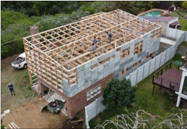
Figure 4: Winbau house under construction
