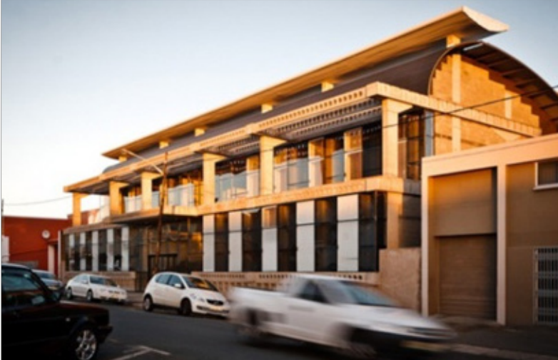
Figure 5: University of Fort Hare, New Complex north façade
