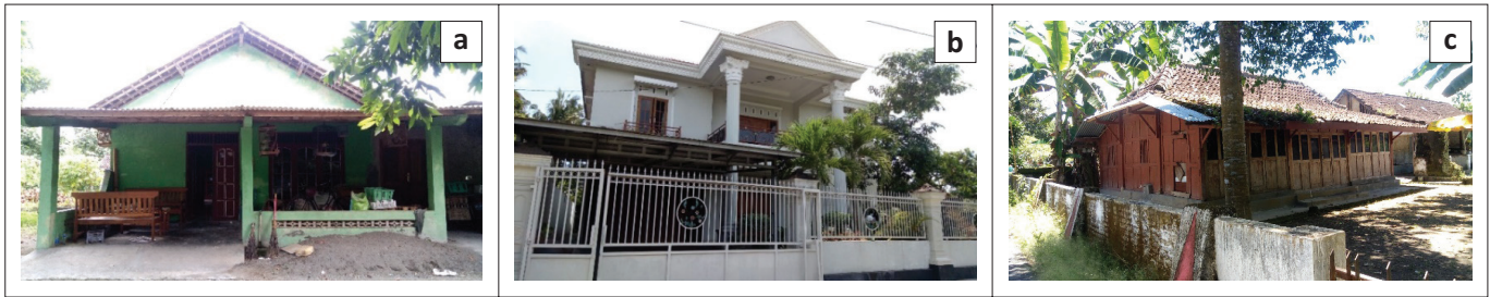
FIGURE 4: (a) Sample of confined masonry, (b) sample of reinforced concrete medium rice frame with masonry infill walls and (c) timber frame.
