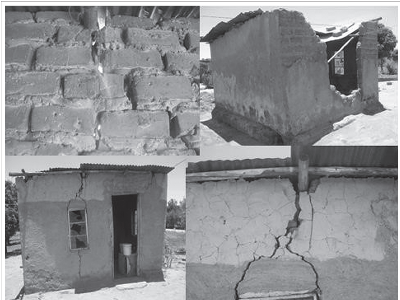
FIGURE 2: Collapsed houses and cracks in Hamutsha-Muongamunwe village.
