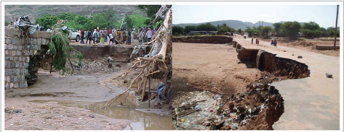
FIGURE 3: Damage caused by 2006 floods on Dachatu Bridge and the road.
