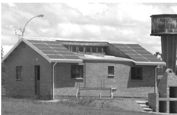
Figure 3: The energy efficient BIPV house
