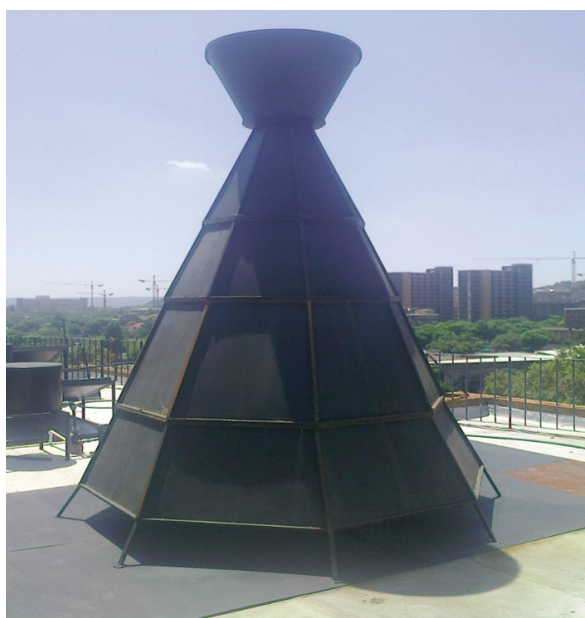
Figure 10: The completed constructed pilot plant used in this study.
