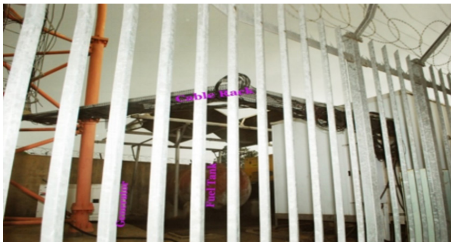
Figure 6. A photo which failed to show the technical layout of the supporting infrastructure at the selected site (Source: EIAR No. 65, 2015, Table 5).
