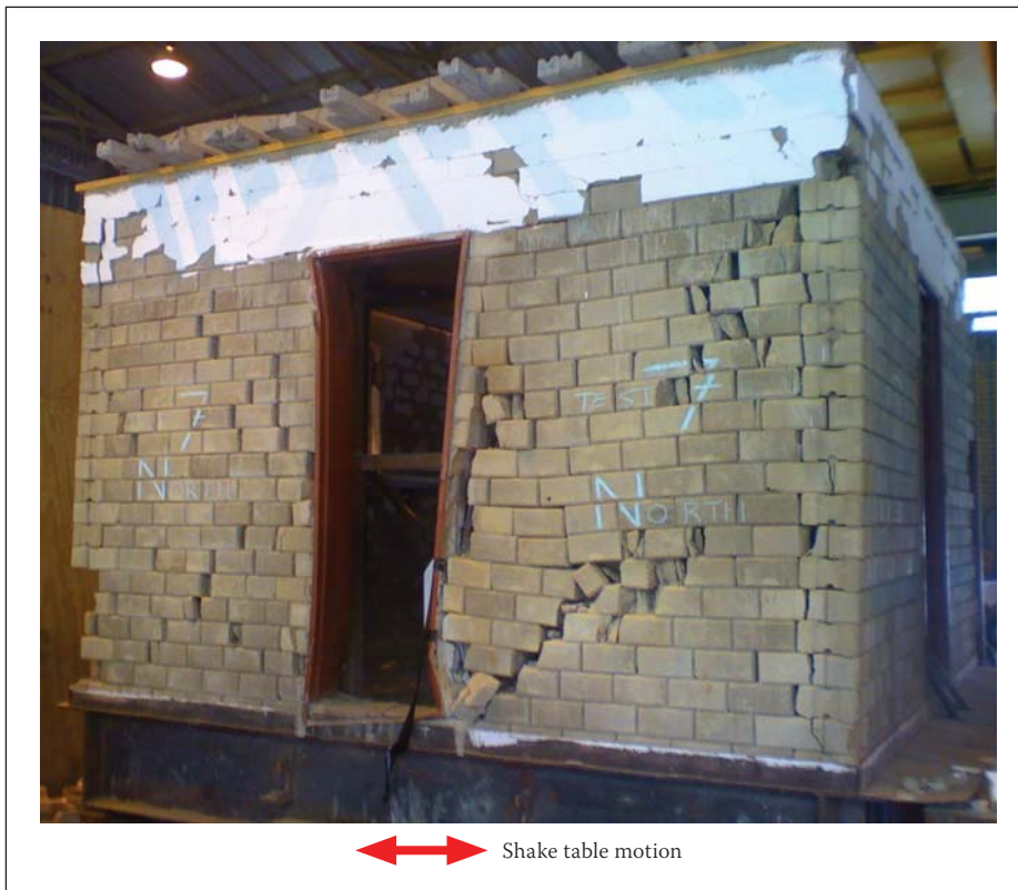
Figure 13 Damaged test structure showing the north wall after the base had been subjected to a 22 mm, harmonic 3 Hz motion for 15 seconds
