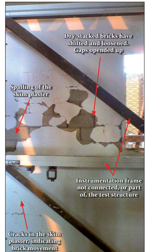
Figure 7 Partial spalling and cracking of the skim plaster on the south wall of the test structure after the first filtered Llolleo earthquake was applied. The view is from the inside of the test structure
