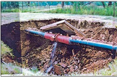
Figure 5 Effect of broken sewer on formation of sinkhole (Pretoria, South Africa)
