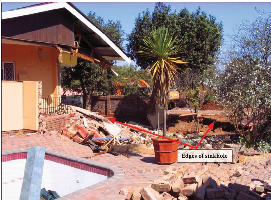
Figure 3 Sinkhole in residential infiltration regime (Centurion, South Africa)
