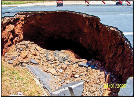
Figure 12 Typical capping of road pavement over sinkhole (Centurion, South Africa)
