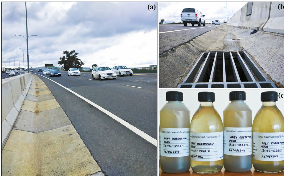
Figure 2 (a) Highway sample location, (b) catchpit inlet, (c) runoff samples
