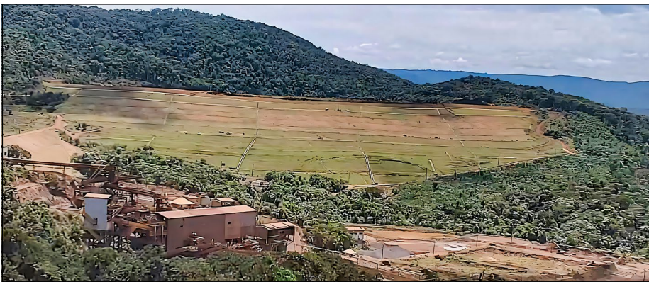
Image 2 Image of Brumadinho at onset of failure initiation (25 January 2019)
