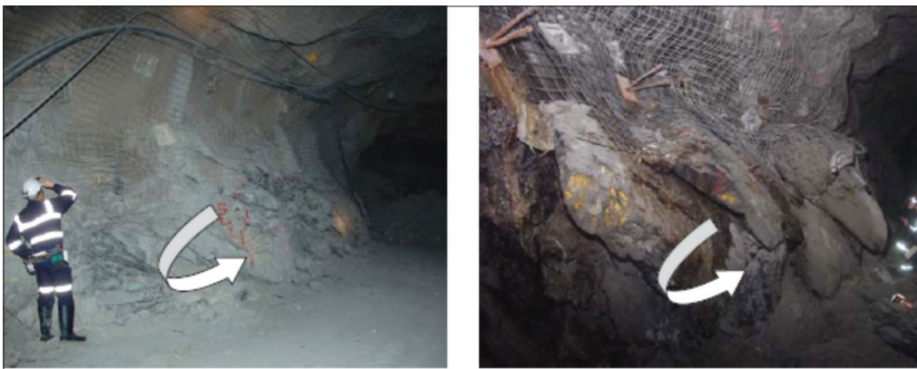
Figure 6—Footwall slabs rotating upwards
