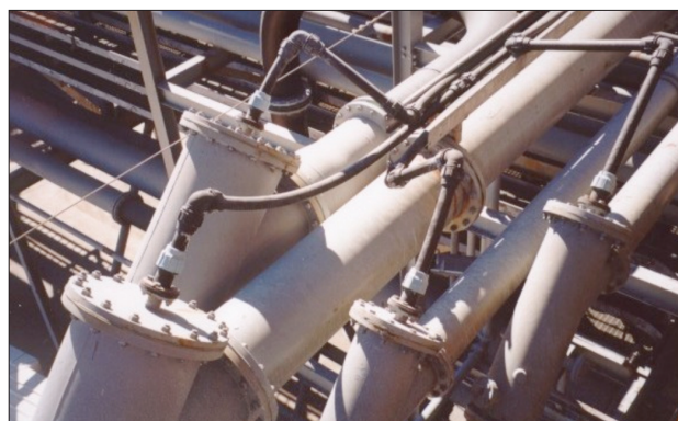
Figure 16—Pressure pipe samplers do not extract a full cross-section of the slurry stream, so the samples taken are unreliable
