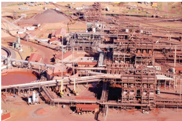
Figure 5—Washing, screening, jigging, and cyclone plant at Parsons
