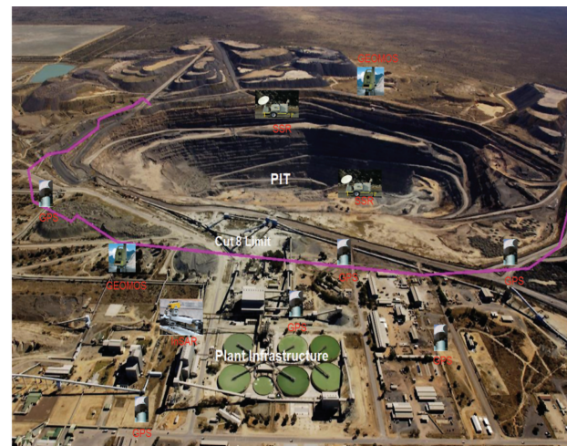
Figure 6—Monitoring equipment positioning
