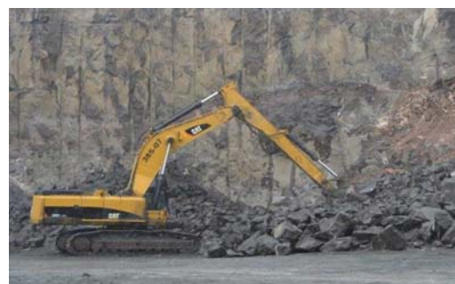
Figure 5—Scaler working on highwalls
