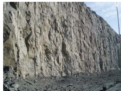
Figure 3—Single-pass 28 m pre-split on basalt
