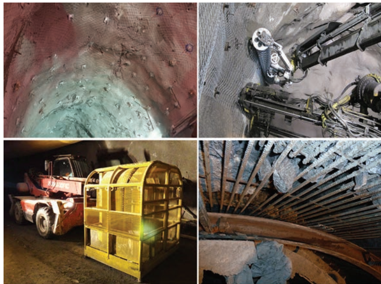
Figure 19—Risk management tools for rockbursts in tunnels (clockwise from top left): layered support with redundant energy and retention capacity to maintain safety in the event of dynamic rupture; robotic bolting and mesh installation to reduce worker exposure; a rock retention and worker protection system for TBM drives; and a multi-function cage for work at a tunnel face or under incomplete support
