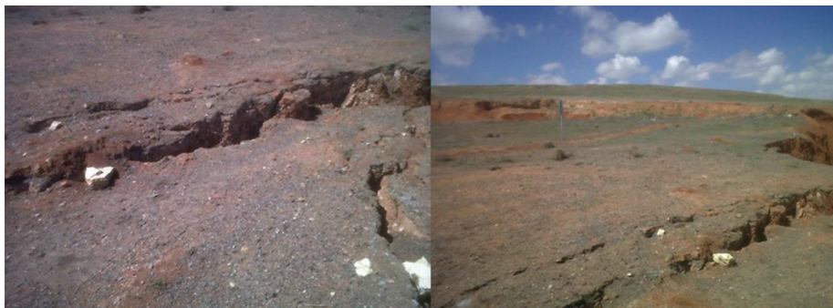
Figure 1 – Tension cracks formed in the field
