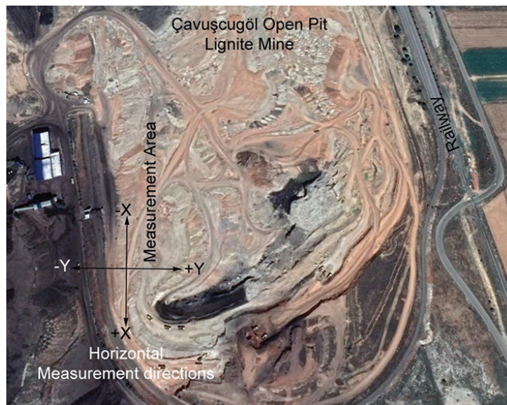
Figure 2b—Plan view of the open pit and the horizontal directions defined in the measurement system for monitoring movements on the tension cracks
