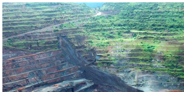
Figure 4—Open pit after failure (March 2017)
