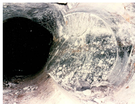
Figure 3—Exposed face of a stope corer hole
