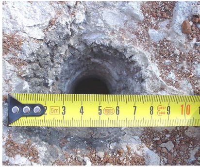
Figure 5—Hole diameter expansion from 32 mm to 40–50 mm with a shattered zone of ~ 80 mm
