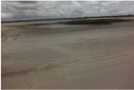
Figure 3—The tailings dam storage facility at Nampundwe mine
