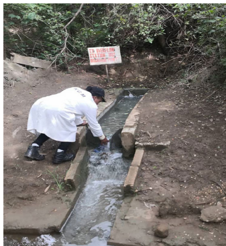
Figure 8—The decant or the overflow from the mine tailings storage at Nampundwe mine
