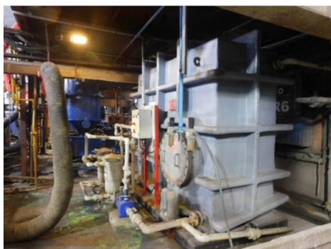
Figure 6—Granulation water recycle plant, front and back view
