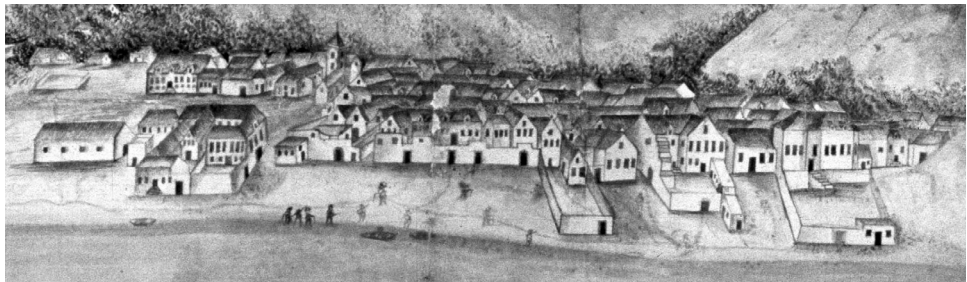
Figure 2: (a) E. V. Stade's view of Table Valley from Table Bay, 1710, and (b) an anonymous view of about 1730. The large houses to the left of the church and facing the shore show features associated with the Dutch double house and heerenhuis styles. (Algemeen Rijksarchief Topo 15-86; Museum Afrika)
