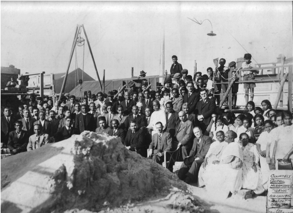
Figure 1: Laying the foundation for a new Tamil school in Vrededorp. (Boris Leiboff, 1940)
