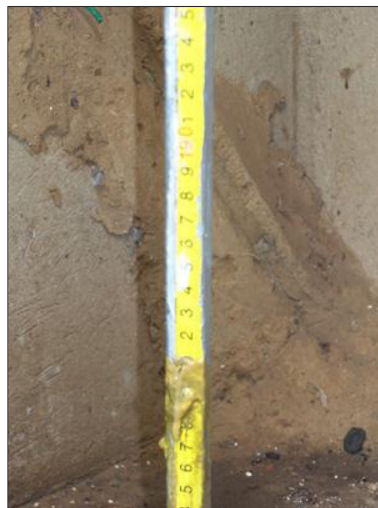
Figure 4 Depth tool with sludge markings (Makerere University, 2015)
